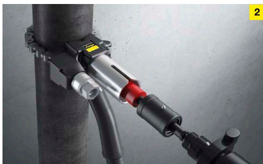
2. Drill the hole with the drilling machine and remove drill guide.
