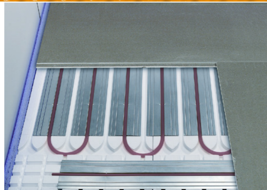
Floor construction with dry screed boards
